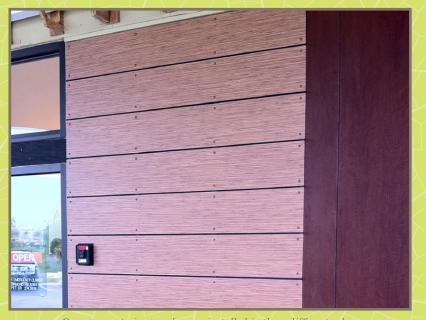
Over 241 exterior panels were installed in three different colors, attached with metal screws to match panels.
