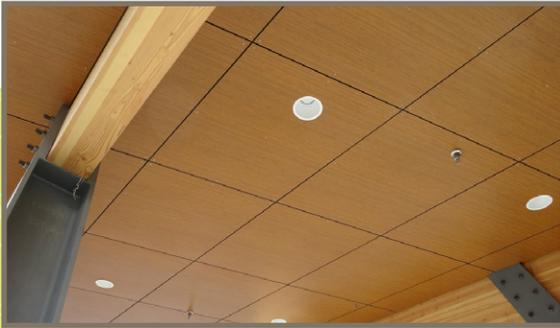
*Stonewood Architectural Panels in Asian Sun were attached to gypsum and steel deck using stainless steel screws.*
