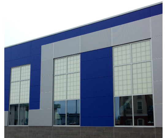
Durable Stonewood Architectural Panels installed to replace damaged competitor panels on the exterior of the Covenant House in Anchorage, Alaska.
