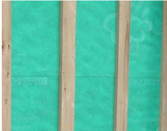
Roofshield/Vaproshield Water Resistant Barrier Application under pressure treated vertical strapping
