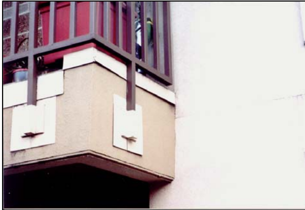
Typical Balcony Corner and Railing Attachment Before Inspection
