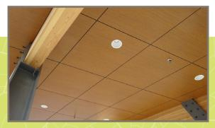
Stonewood Architectural Panels in Asian Sun were attached to gypsum and steel deck using stainless steel screws.
