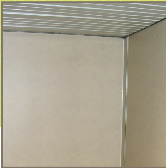
Multiple panels at the end of the jet bridge create uniform seams and are easy to clean.
