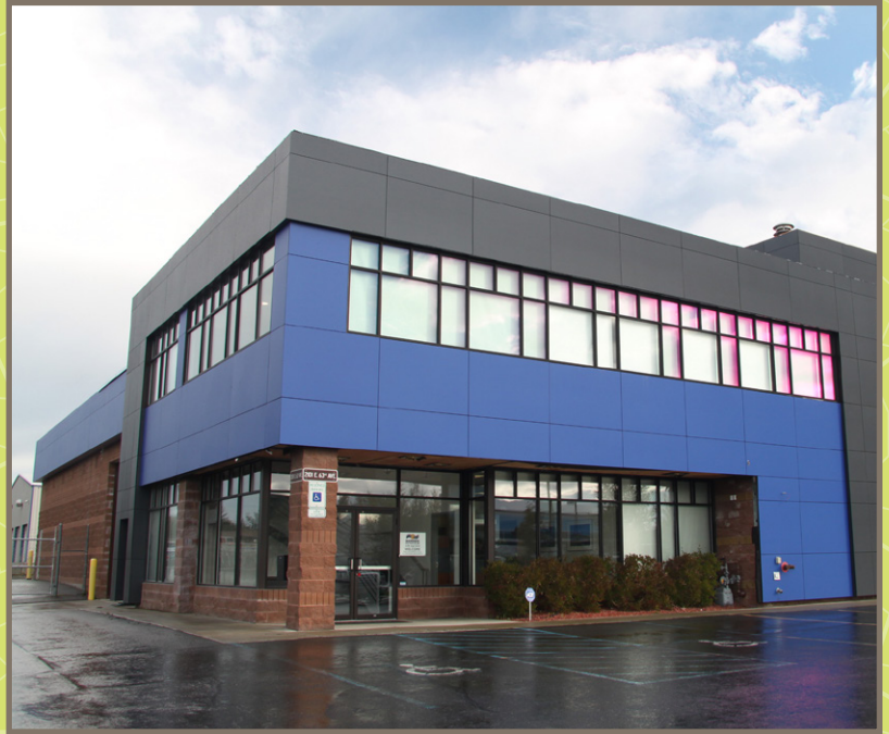
Carbon Mesh and Lapis Blue Stonewood Architectural Panels were installed on the Shoreside Petroleum Inc. terminal in Anchorage, Alaska.
