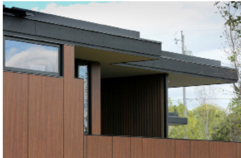
Though the panels are made in 4-by-8-foot sheets, the architect used alternating widths to enhance the visual interest of the building, and was also able to cut the panels on site.
