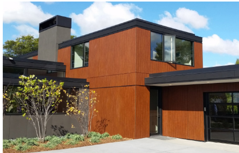
Though the panels are made in 4-by-8-foot sheets, the architect used alternating widths to enhance the visual interest of the building, and was also able to cut the panels on site.
