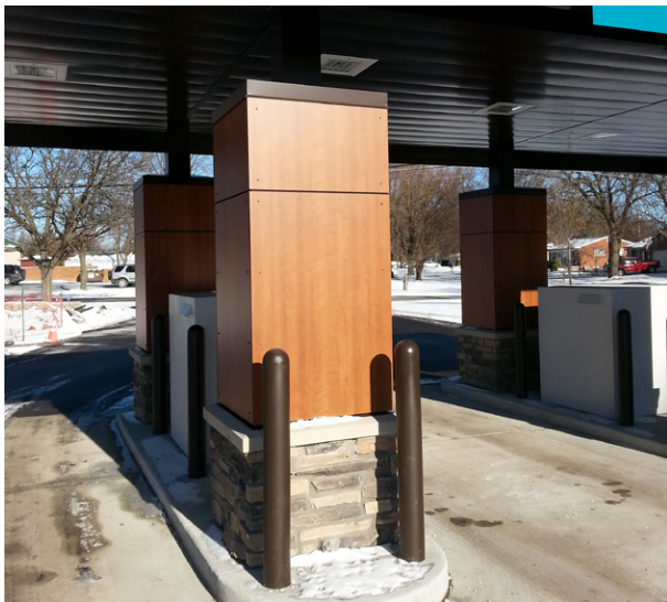
Colored fasteners were used to enhance the building's vibrant exterior.
